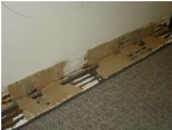
This is an area of fungal growth on the south wall of room 90 C. The Dark IR image on the left indicates an area of elevated moisture.
