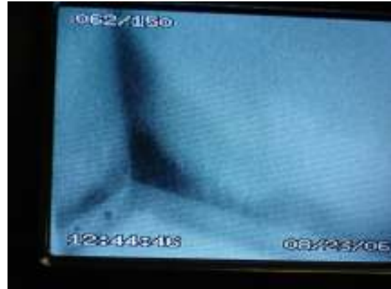
Room 90C Northwest corner – Area of water damage. The dark area on the IR photo has elevated moisture levels.
