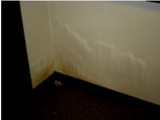
Room 90C Northwest corner – Area of water damage. The dark area on the IR photo has elevated moisture levels.
